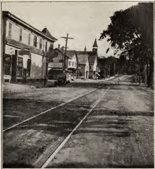
Main Street, Showing Need of Widening
